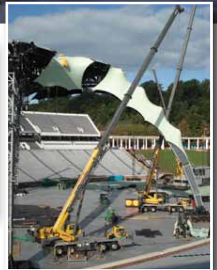
To erect the stage W. O. Grubb used two Liebherr LTM-1060/2s, a Grove TMS-900E and a Grove TMS-800E
