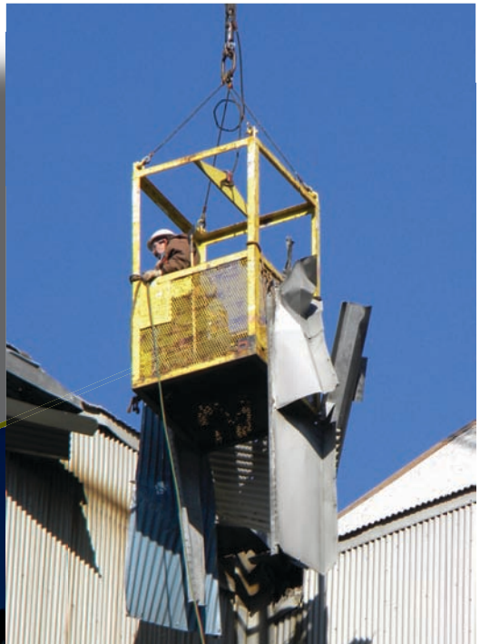
Official inspecting the damage in the personnel basket hoisted by the Demag AC 140
