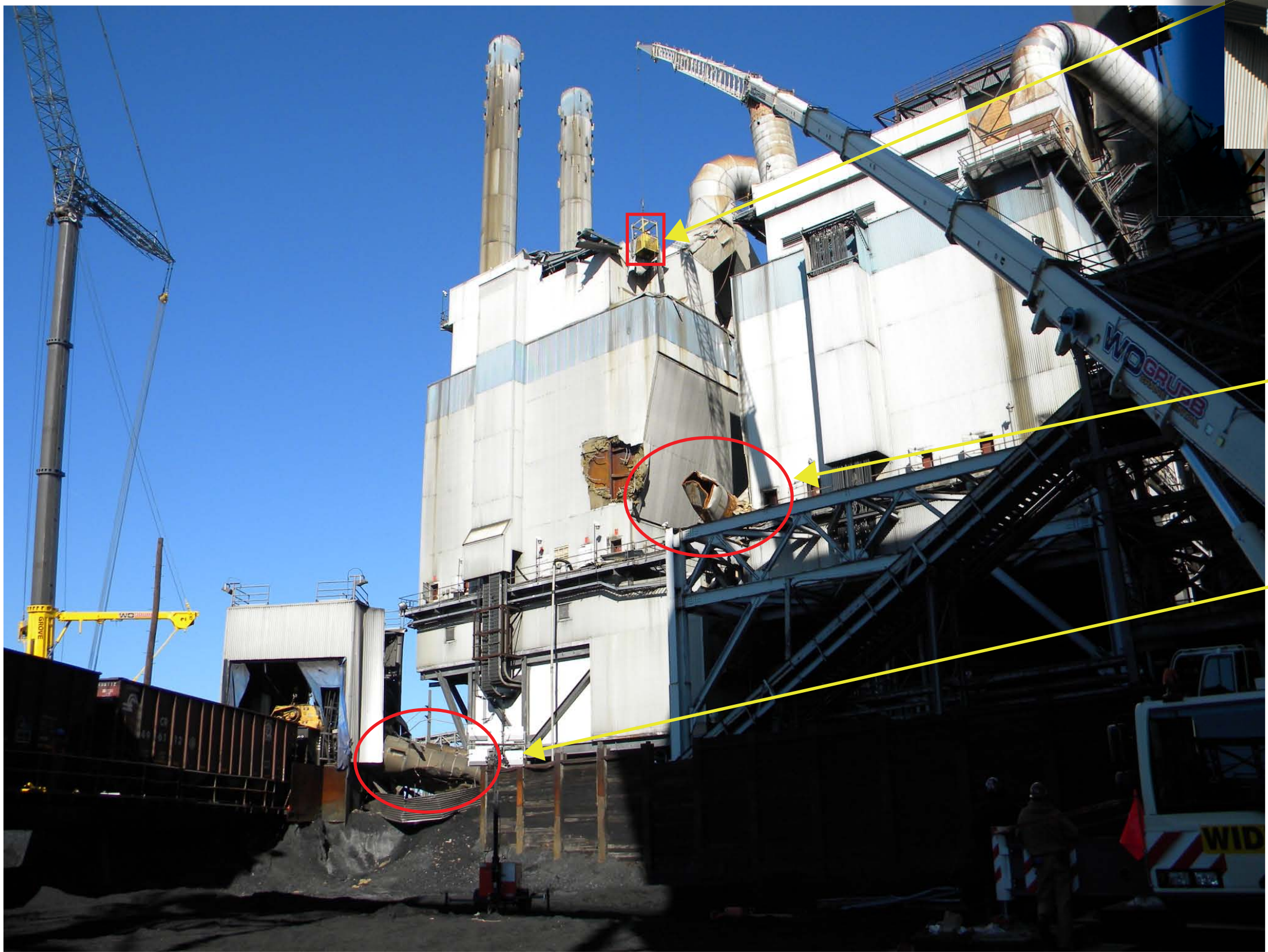
Official inspecting the damage in the personnel basket hoisted by the Demag AC 140
